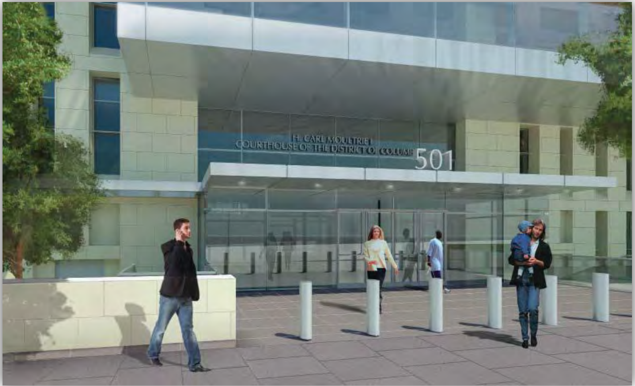
C Street Expansion Entry
