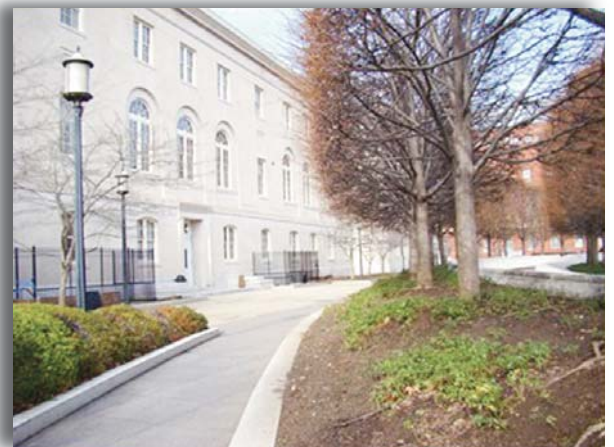
Building A park side entrance.
