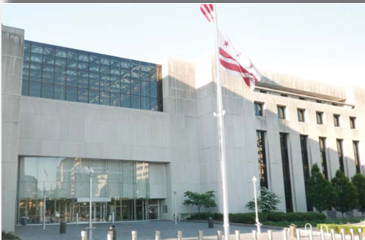
Reconfigured Moultrie Courthouse main entrance.
