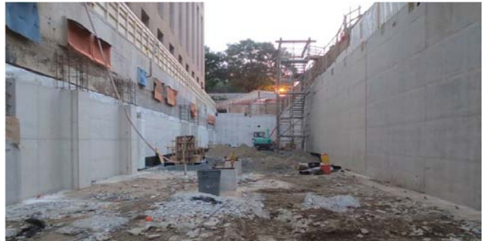
Moultrie Courthouse Addition Foundation Takes Shape.
