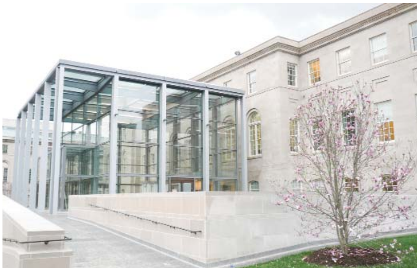
The Historic Courthouse's new entry.
