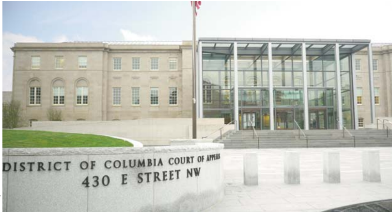
The new front of the Historic Courthouse, a National Historic Landmark and one of the oldest public buildings in the District of Columbia. Photo by Dennis Shipley
